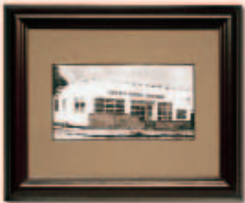
The Credit Union Building at Broadway and Quebec, where VanCity operated during its early years.
